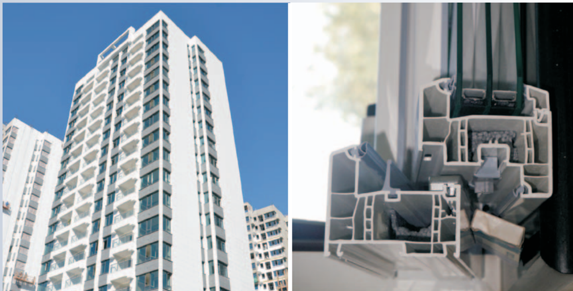
Figure 18: Chinese near-zero-energy residential high-rise building and high-performance windows
