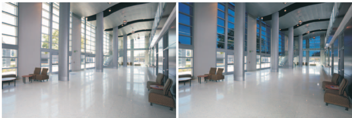
Figure 4: Large-scale demonstration of electrochromic glazing at Chabot College, California
